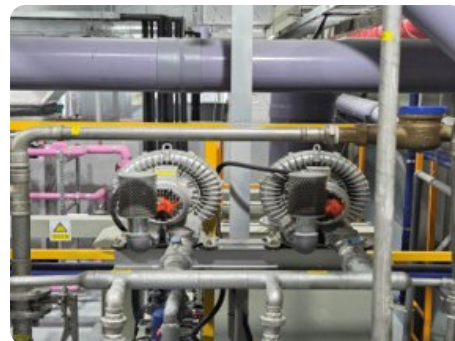
Installation of Additional Ring Blowers in the Wastewater Treatment Plant
